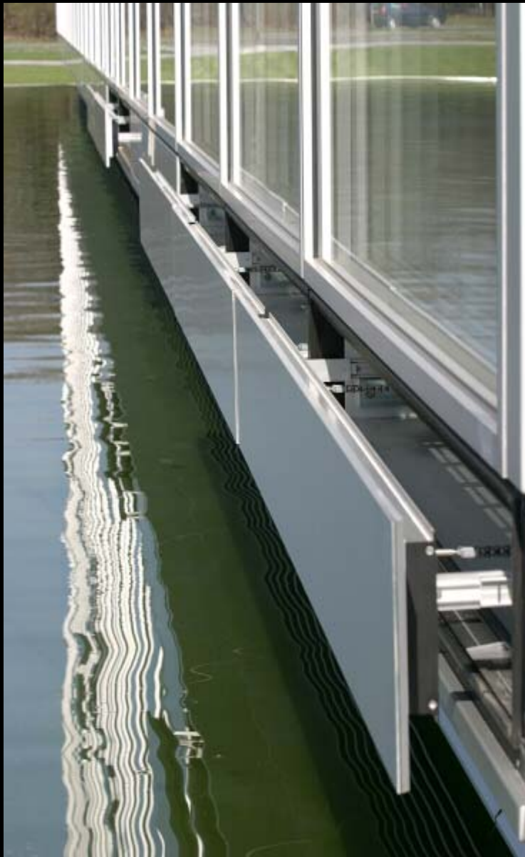
Facade integrated ventilation - custom built
